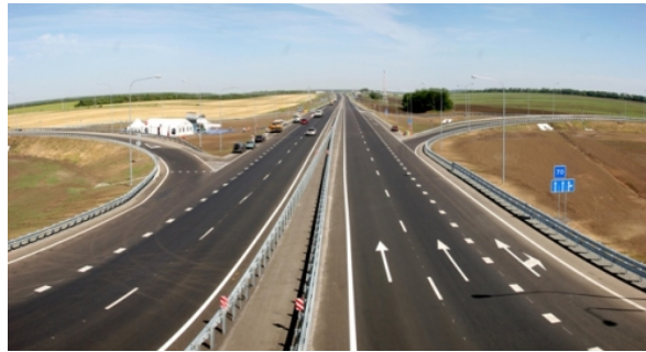
Figure 9.2: Figure 9.2 Highway with a median that divides the road in half [2]
